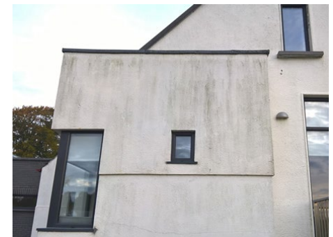
Render that has become unattractive due to staining
