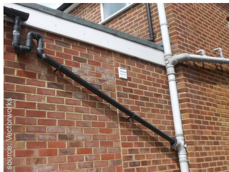
Drain pipes not designed in from the start are likely to detract from the facade
